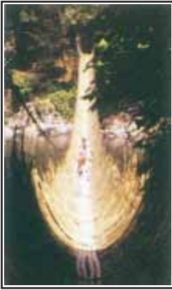
Figure 6.7 : Rope Bridge (Arunachal Pradesh)
